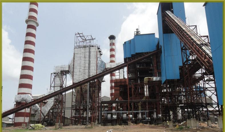
Project Site: M/s. Jamkhandi Sugars Ltd. India (Karnataka) Boiler Capacity: 90 TPH X 72.4 Kg/Cm<sup>2</sup> Traveling Grate Fired Boiler
